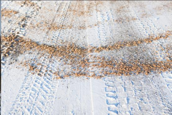
Salt is spread over icy road surfaces. The salt helps the ice to melt.
